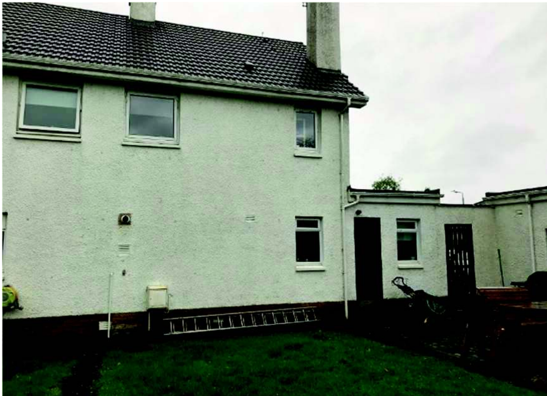
11 Rear of vestibule towards garage
