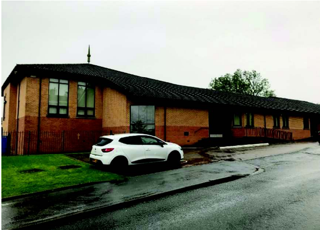
1 Main entrance and sanctuary
